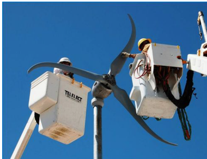
Figure 6. Maintenance of a Wind Turbine
