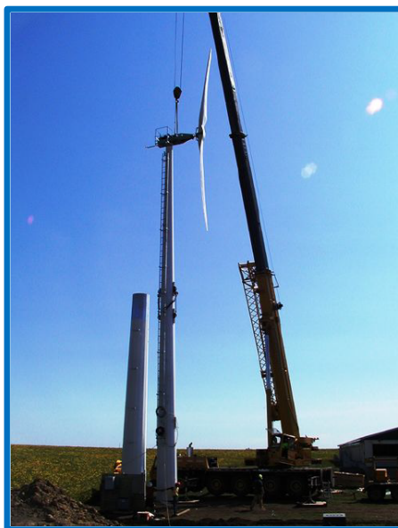
Figure 7. Installation of a Wind Turbine
